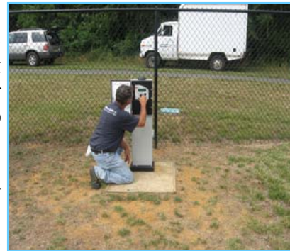
Installation of a Smart Controller at Thompson Park Soccer Field in East Greenwich Twp., NJ
